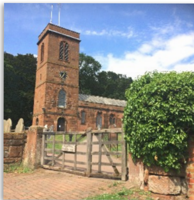
The Dilapidated Gates Are Being Replaced
