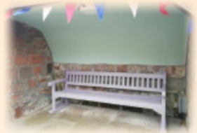
Refurbished bus stop
