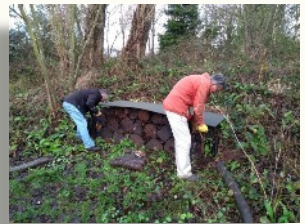
Putting on the Roof
